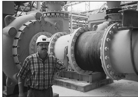
A 40" (1016mm) diameter series 100 hose installed in the suction line, drawing river water into condenser cooling service.
