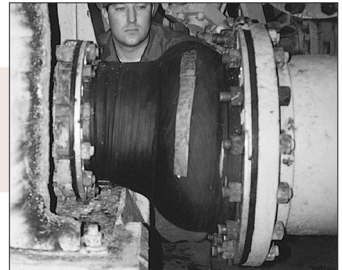
Measurements being taken for a retrofit. The eccentric reducer was manufactured to the exact length with non-parallel flanges. The photo at right shows the reducer after installation.
