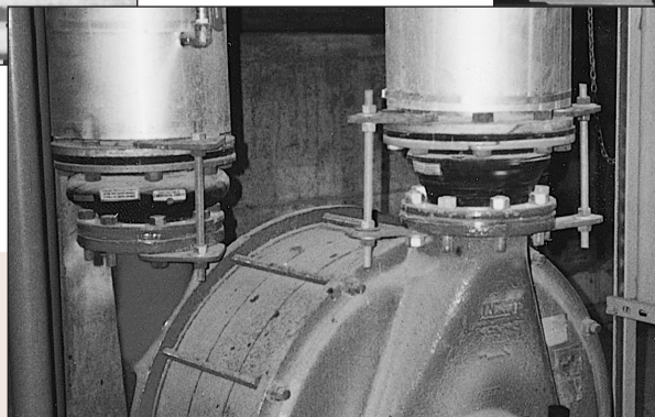
Concentric reducers installed in the suction and discharge air connections of a positive displacement high pressure blower, reduce stress to the flanges and facilitate hook-ups.
